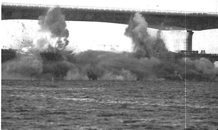
Second of two in-air explosions to demolish the bascule sections of the old Ringling bridge. A portion of the new Ringling fixed-span bridge can be seen in the background.
