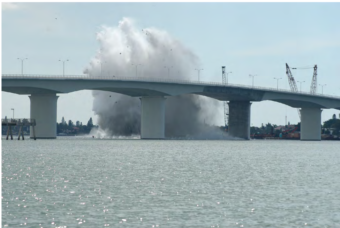
FIG. 7 Demolition of previous bridge supports during construction of new bridge in Sarasota Bay in 2003 (Buckstaff et al., 2013).
